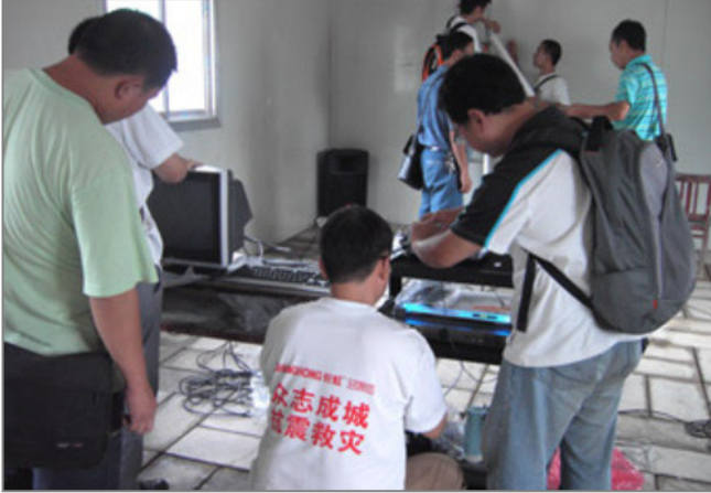
Installation workers testing the equipment
